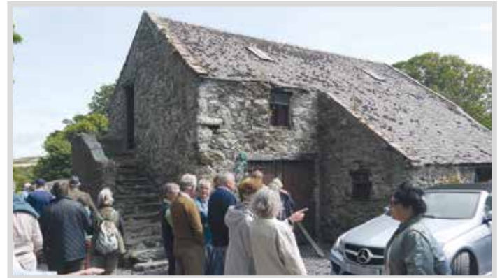
Dronwy stable block with exterior staircase
