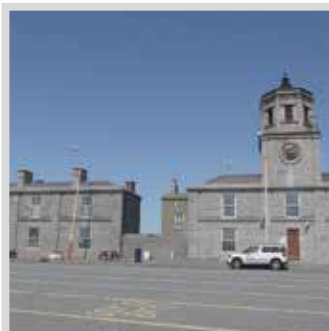
Telford's Clock House and Customs office
