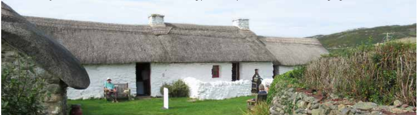
Swtan, Church Bay
