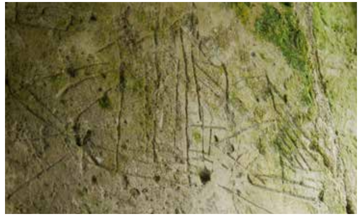
Hafoty: Graffiti on plaster
